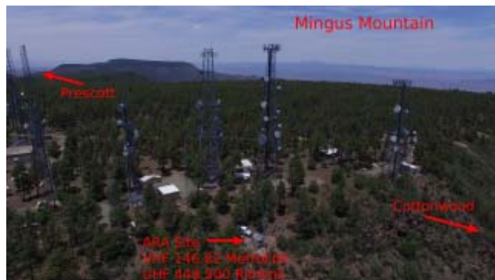
ARA Mingus Tower Annotated
